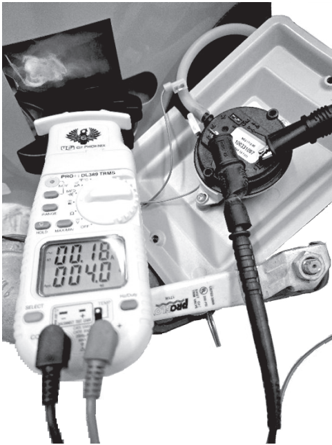
Figure 6. Blocked Exhaust Switch Test
