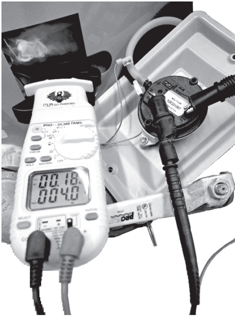
Figure 12. Blocked Exhaust Switch Test
