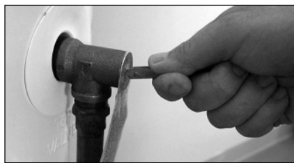
Figure 44 - T&P Relief Valve.
