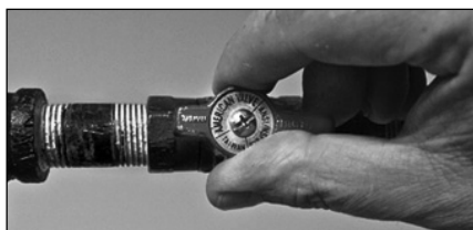
Figure 33 - Gas valve in "on" position
